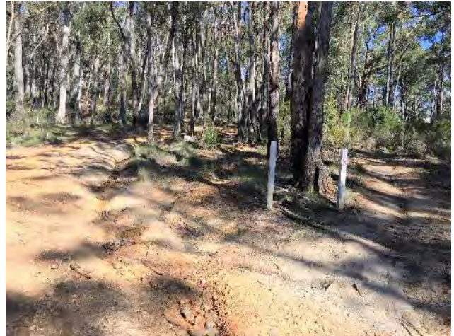
Figure 2. Example of poor emergency track access that should be upgraded to improve trafficability
